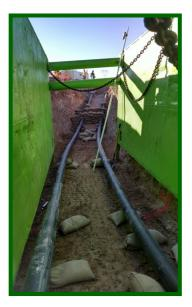
Tiffany crews installed 22,000 lineal feet of 6" HDPE SDR-17 including 10 manholes containing air release valves and two cast-in-place vaults. The new sewer line spans under numerous drainage ditches and washes as well as crossing various roadways by either open cut or directional drilling before reaching a new sewage treatment plant built at the Water Reclamation Facility.
