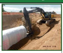
TCC Crews successfully completed the PVNGS Fall Outage at the end of October. This outage involved the excavation, repair and backfill of 18 spools within 12 days.
